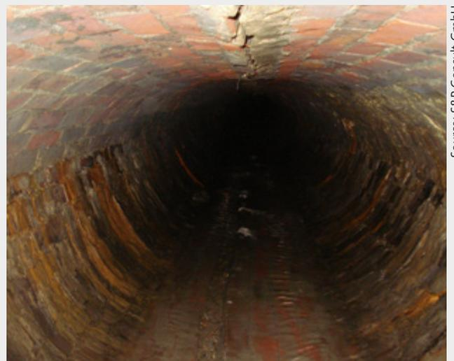
**Figure 5:** Significant longitudinal crack in the crown and in the invert, heavily deformed cross-section
