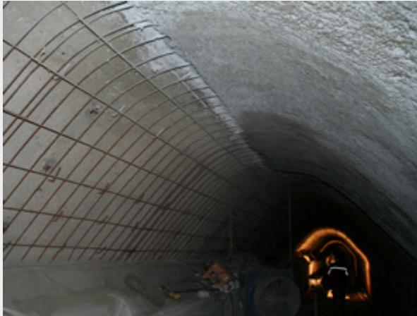
Figure 9: Reinforcement of the shotcrete shell
