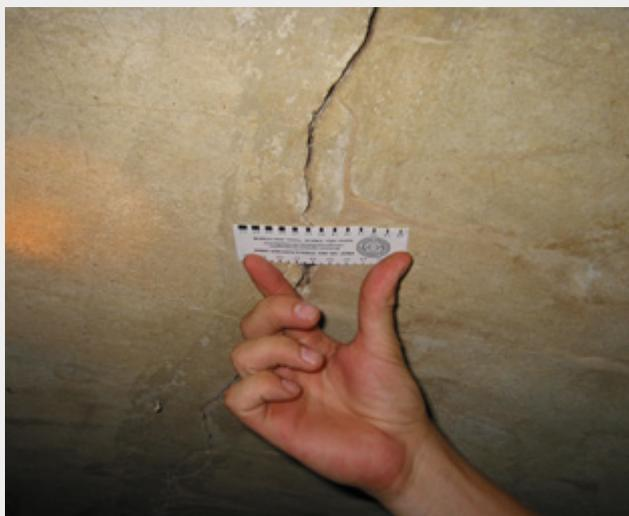
**Figure 4:** Longitudinal crack in cast-in-place concrete sewer, source: S&P Consult GmbH
