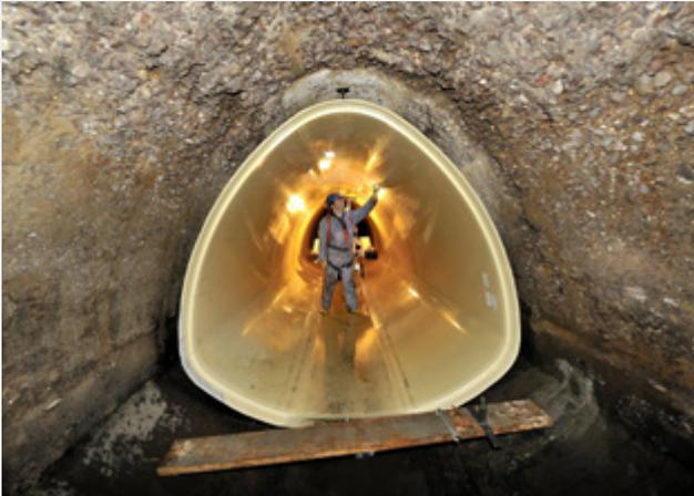
**Figure 6:** GRP short pipe lining, source: HOBAS Rohre GmbH
